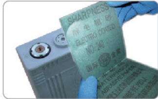
Battery terminal pole sanding
